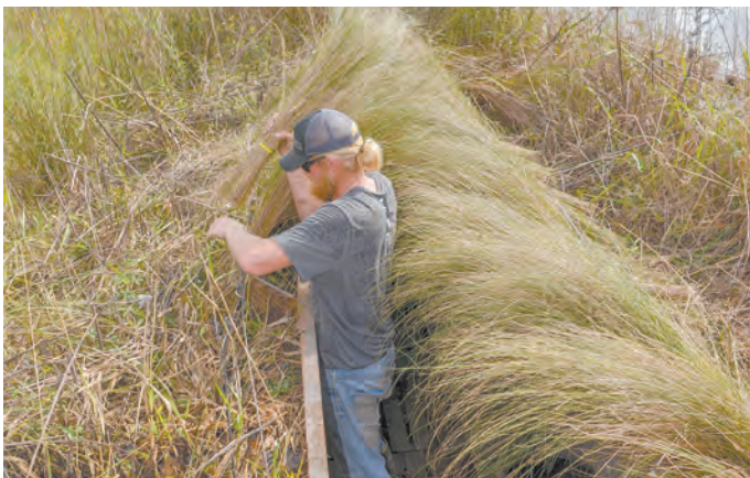
6. Working from inside the blind to preserve as much natural vegetation as possible, salt grass bundles are inserted between the stretched bungees and the livestock panels.
